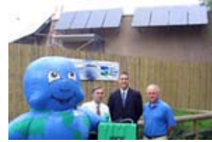
Houston Zoo Solar Installation
